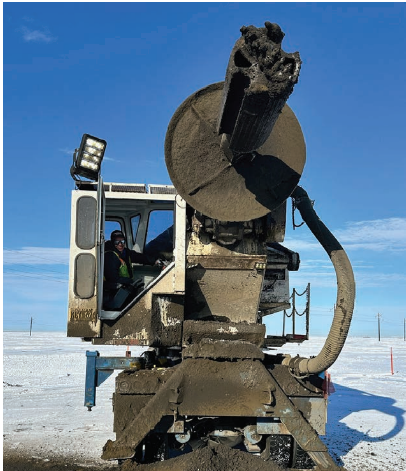
Apprentice Steven Sparks in Doyon's Watson drill at Santos' Pikka project on the North Slope; Steven is drilling holes for Vertical Support Members (VSM); pipe is elevated instead of buried because the pipe would thaw the permanently frozen soils of the tundra; photo courtesy of Local 302 member Benjamin Johnson
